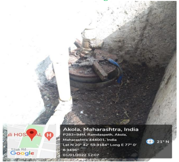
Bore Well near Girls Hostel
